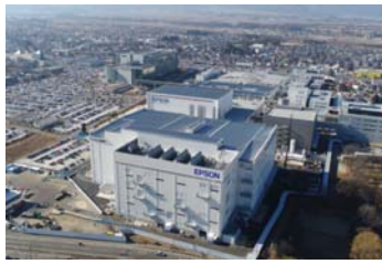
New plant (Building 9) at the Hirooka Office
