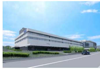
Innovation Center Building B in Hirooka (under construction)
